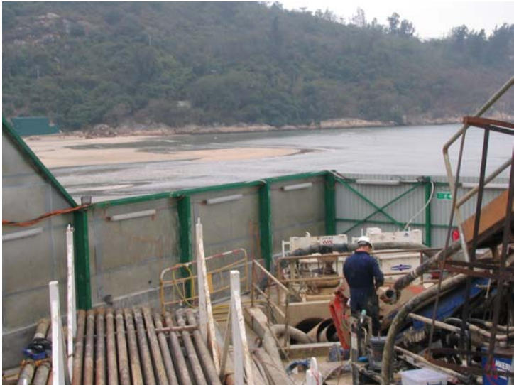
HDD Site at end of Chi Ma Wan Tunnel
