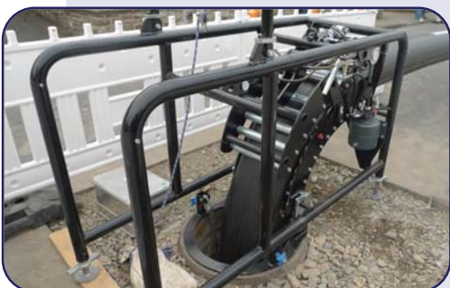
Burstform in operation using the advanced QuickLock rod technology
